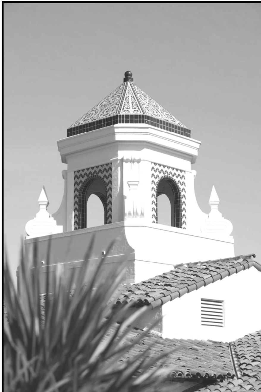
View of City Hall from the parking structure near the new Main Library.
